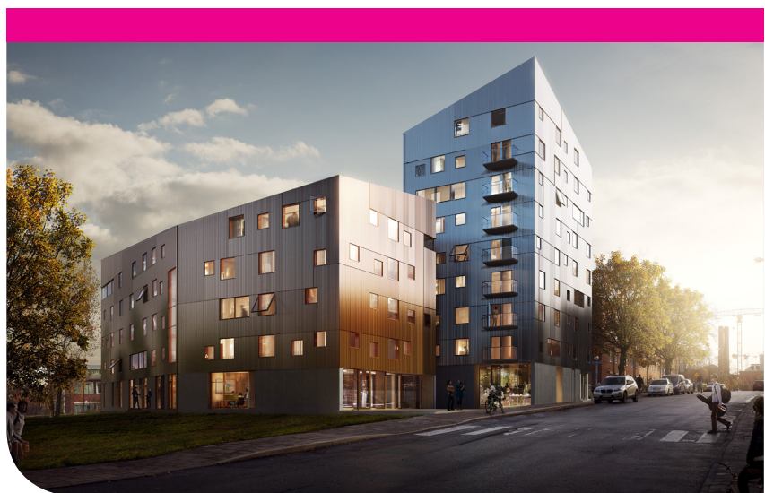
Construction of 600 student housing units on the Royal Institute of Technology Campus Architect: Utopia arkitekter / Main contractor: ByggVesta
