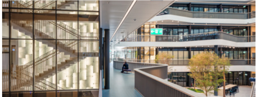
Biomedicum, one of the largest research labs in Europe, was completed for Karolinska Institutet in 2018. This construction project – the largest ever undertaken by Akademiska Hus – was completed ahead of schedule and under budget.
